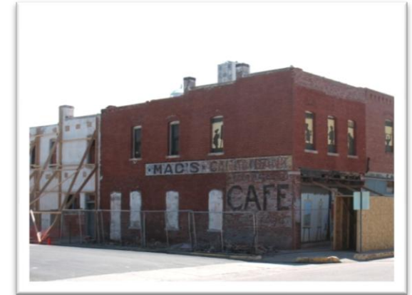
Progress on the Murdock Building exterior restoration, April 2011
