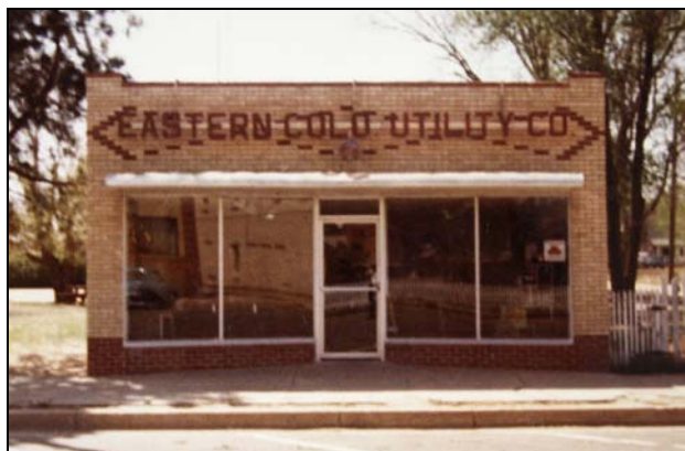
Figure 38. George D. Crow and Joseph Schmitt built this office for their Eastern Colorado Utility Company in Eads in the 1950s. SOURCE: Kiowa County Assessor, old appraisal card photograph, undated.
