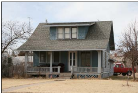
1000 Goff Street, Eads, 5KW.174, Glau House (1907)
