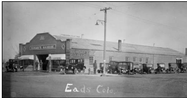
Figure 13. In 1917 Ford dealer Howard R. Sunday built this large garage in Eads at 1111 Maine Street. Today's Crow's Stop 'N' Shop operates in the building. SOURCE: Eads High School, photographic collection.
