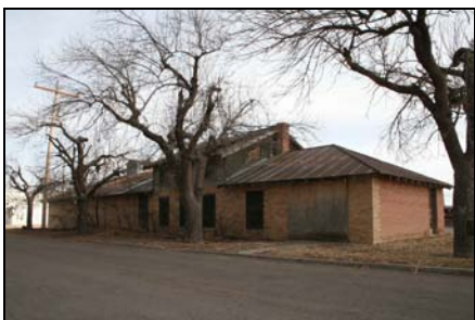
E. 14th Street and Hickman Street (southwest corner), Eads, 5KW.90, Eads Electric Light Plant (Highland Utilities), Southeast Colorado Power (1931)
