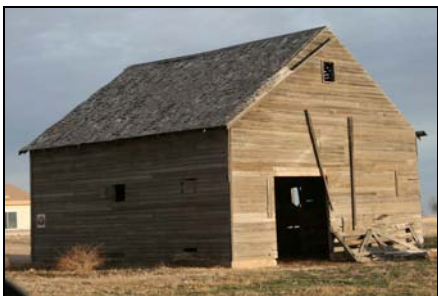
W. Lowell Avenue and S. Slater Street (southeast corner), Eads Vicinity, 5KW.184, Jackson Barn (1915-20)
