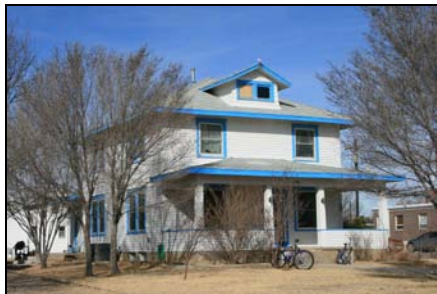
1300 Luther Street, Eads, 5KW.185, Cherry House (1918)
