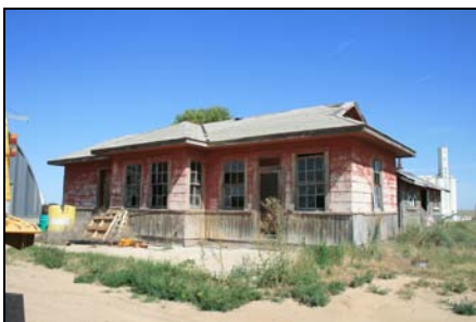
4th Street (south side, two blocks east of Spencer Ave.), Haswell, 5KW.200, Haswell Missouri Pacific Railroad Depot (late 1940s)
