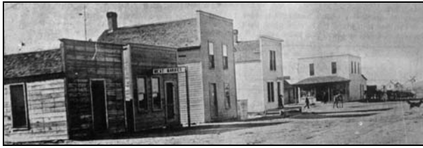
Figure 18. The west side of Main Street in Haswell exhibited examples of false front construction, including the Post Office (the white false front building just right of center), in this late 1910s view. SOURCE: Kiowa County Historical Museum, photographic collection.
