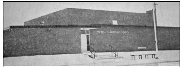
Figure 39. Denver architects Wheeler and Lewis prepared the plans for the 1963 Haswell Elementary School, which featured a large gymnasium providing students with “hours of fun.” SOURCE: Kiowa County Public Library, dedication brochure, 1964.
