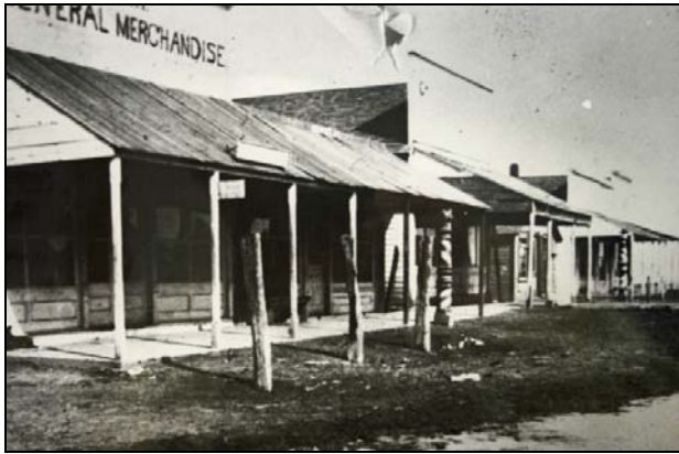
Figure 7. Some of the earliest commercial buildings in Eads and other Kiowa County communities used false fronts to present a more imposing appearance. SOURCE: Kiowa County Public Library, undated, photograph collection.
