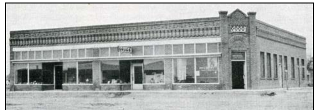
Figure 37. John W. Blair's hardware store occupied the southern storefront in the 1917 Fluke and Blair Building in the 1200 block of Maine Street, Eads. SOURCE: Teal and Jacobs, Kiowa County , 248.
