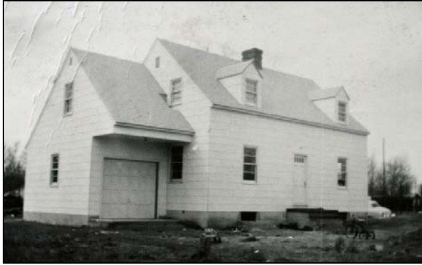
Figure 26. Dr. G. Erle and Ella Moore built this Cape Cod style residence at 1100 Kerr Street in Eads in 1949. SOURCE: Kiowa County Assessor, old appraisal card photograph, undated, c. early 1950s.
