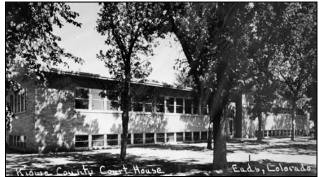
Figure 28. C. Francis Pillsbury of Denver designed the International style 1956 Kiowa County Courthouse. SOURCE: Kiowa County Public Library, undated, photograph collection.
